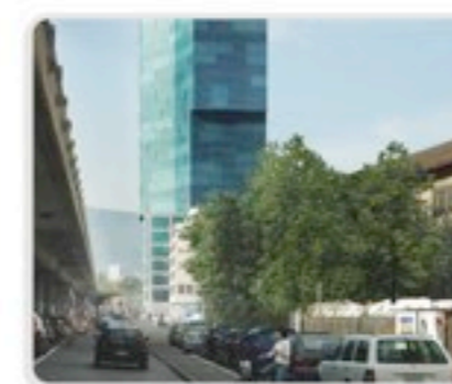
Prime Tower, Schweiz
