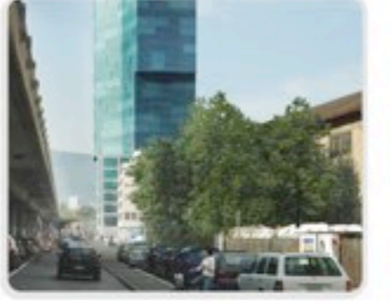
Prime Tower, Schweiz
